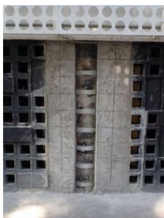
Figure 7 32 - Strengthened post at ground floor level and additional posts
