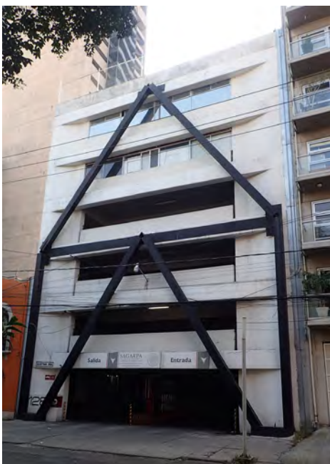
Figure 7 15 - Façade bracing: overall view
