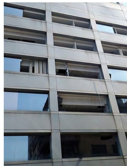
Figure 6 23 - Loss of non-structural glass panels
