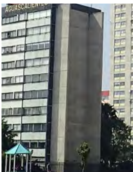
Figure 7 1 - Strengthening using concrete shear panels
