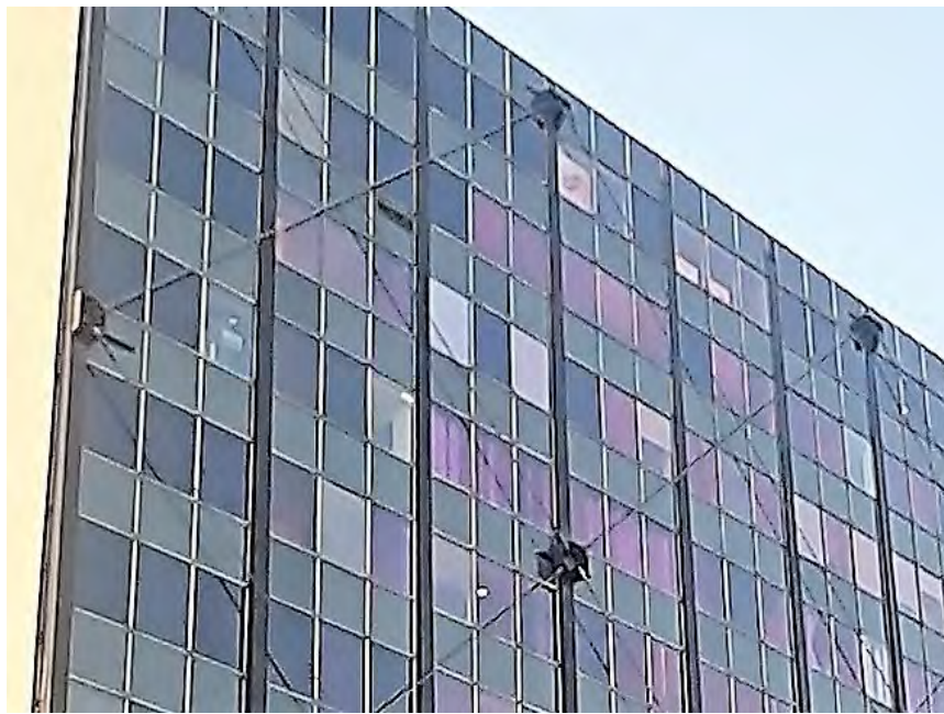
Figure 7-23 - Detail of the metal tie rods
