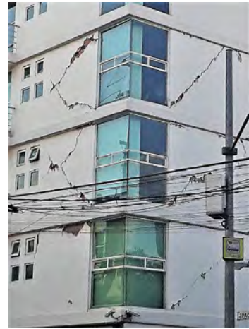
Figure 6 15 - Shear failure of the infill masonry
