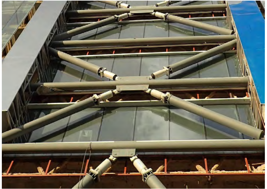
Figure 7-27 - Detail view of the diagonal dampers and horizontal stiffeners
