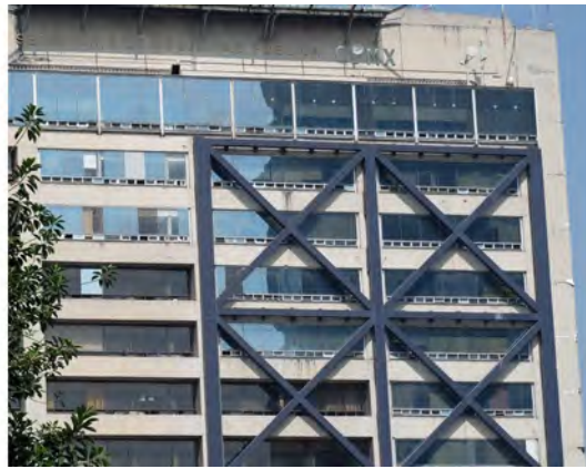
Figure 14.4 – Seismic retro-fitting of buildings after 1985
