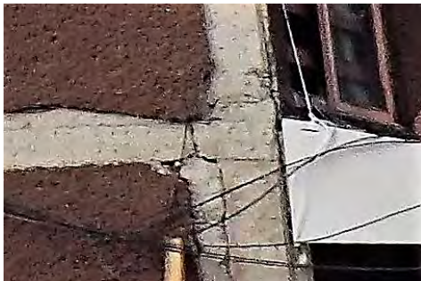
Figure 6 16 - Post-beam junction failure
