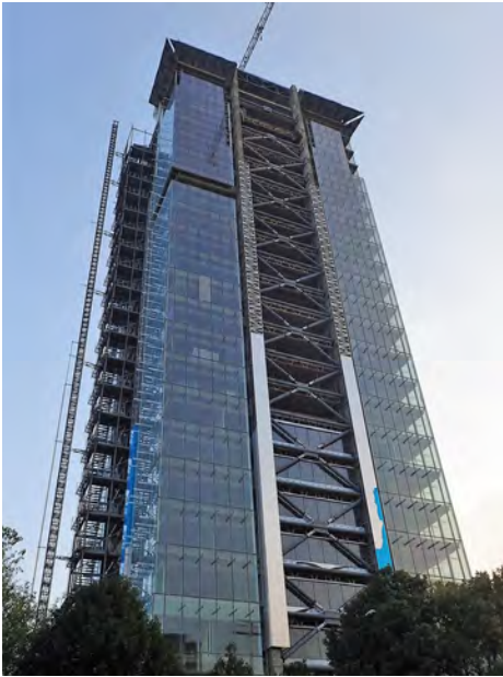
Figure 7-26 - Full height retro-fitting
