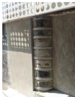
Figure 7 3 - Strengthening of concrete elements
