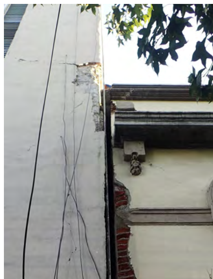
Figure 6 22 - Collision between buildings of different typologies
