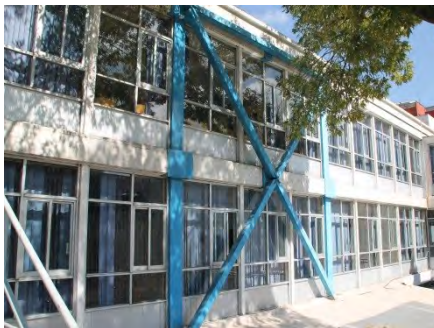
Figure 7 17 - Façade bracing
