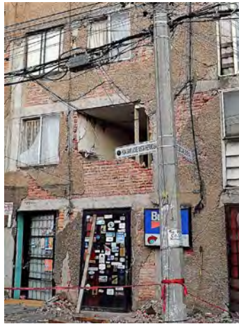
Figure 6 14 - Out-of-plane failure of masonry infill
