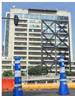
Figure 7 2 - Strengthening using steel braces
