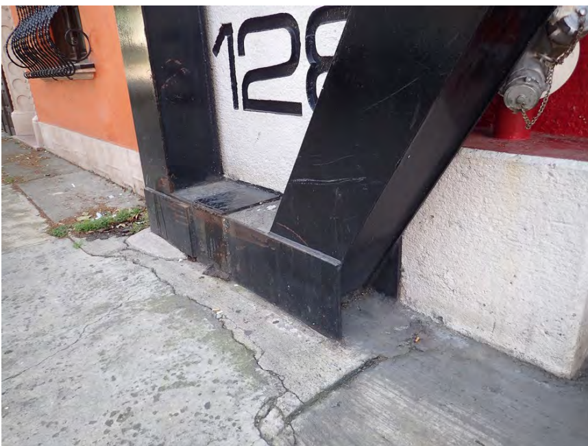
Figure 7 16 - Detail of strengthening at the base of the building
