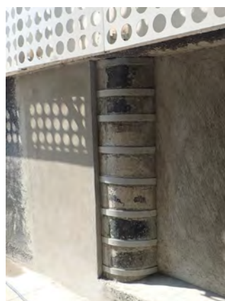
Figure 7 33 - Strengthening of a post
