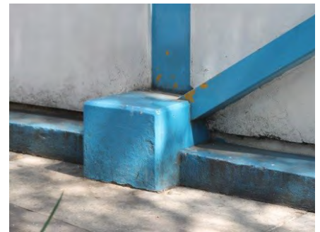
Figure 7 19 - Detail of strengthening at the base of the building
