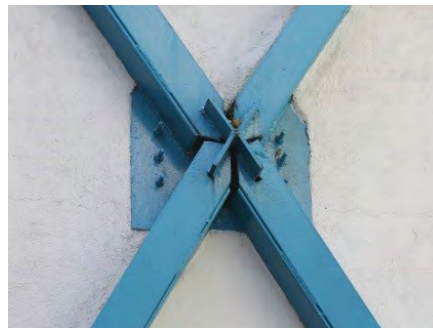
Figure 7 18 - Detail of strengthening system
