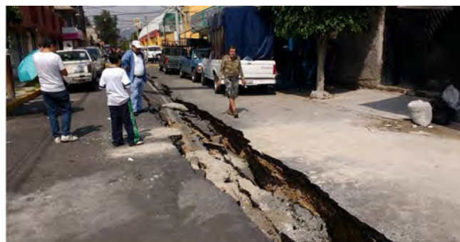
Figure 8.2 – (Pipe repair works in Ixtaltepec (Oaxaca). (Right) Road collapse in Tlahuac (CDMX) due to a damaged water pipe.
