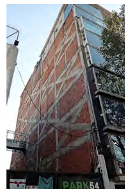
Figure 6 3 - Concrete cross bracing
