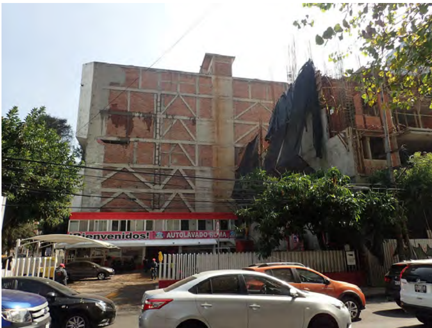
Figure 7 11 - Bracing on a masonry wall
