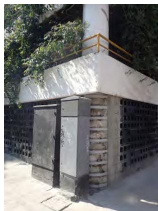
Figure 7 31 - Strengthened corner post and buttress post
