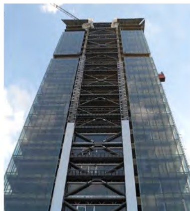
Figure 14.6 – Visually affirmed bracing on recent buildings
