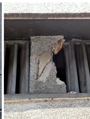
Figure 6 20 - Short post failure
