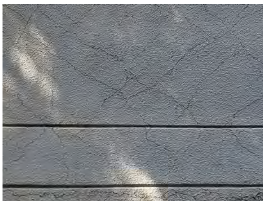
Figure 6 19 - Appearance of the shear crack (detail)
