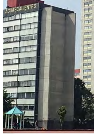
Figure 7 9 - Full-height orthogonal shear walling
