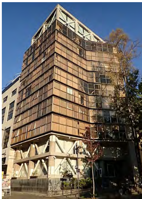
Figure 7 13 - Cross bracing strengthening – overall view
